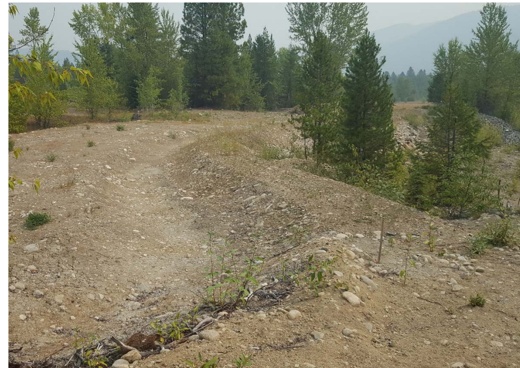
Photograph 4: South TSF, Cell 1, crest and upstream ditch at southeast embankment, looking northeast. 8 August 2017.
