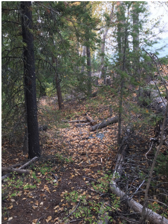
Downstream Side of Cell 3 Dike
