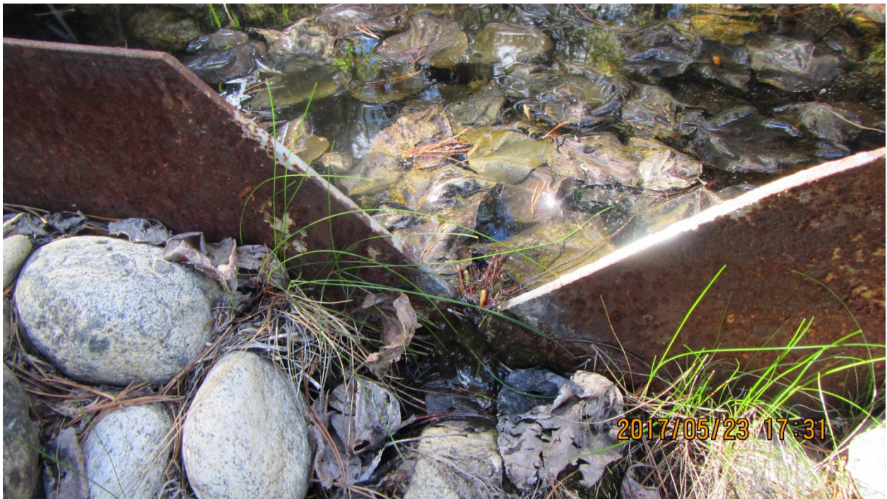
Weir at Decant Outlet Cell 6
