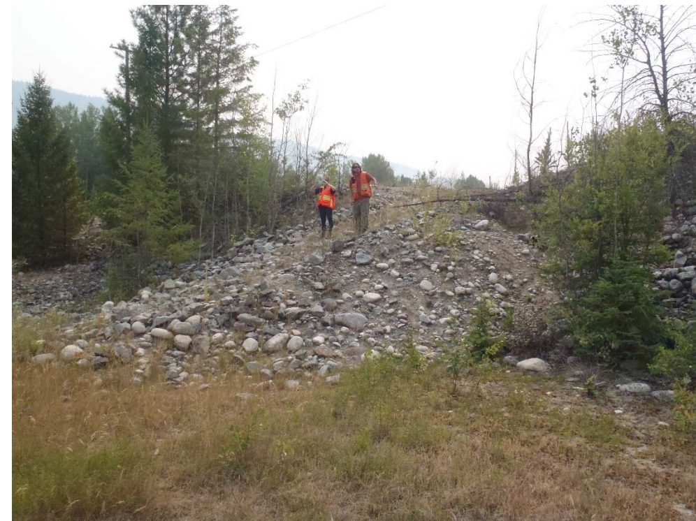
Photograph 23: South TSF, spillway between Cell 4 and Cell 3, looking south. 8 August 2017.
