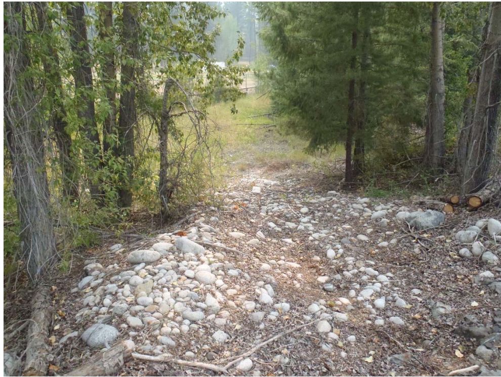
Photograph 27: South TSF, Cell 3, spillway from Cell 3 crest, looking east from crest. 8 August 2017.
