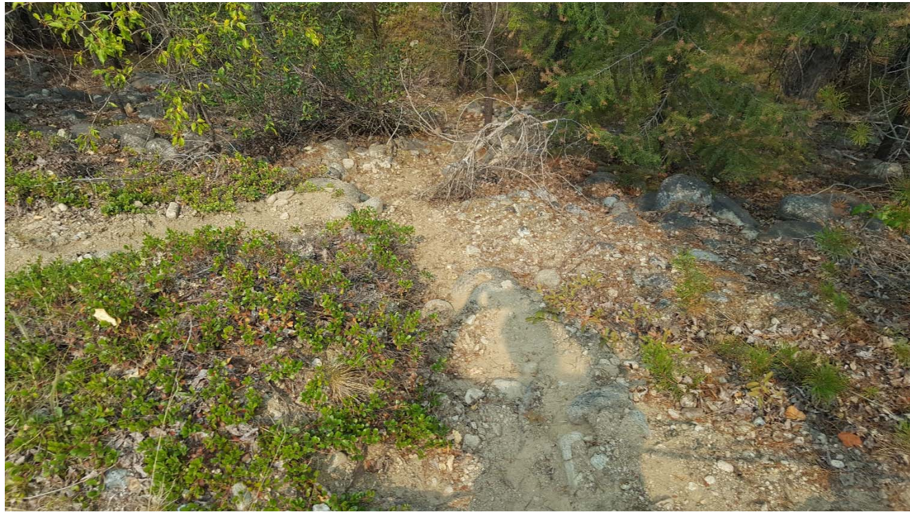
Photograph 37: North TSF, Cell 6, minor erosion on downstream dam slope, looking north. 8 August 2017.
