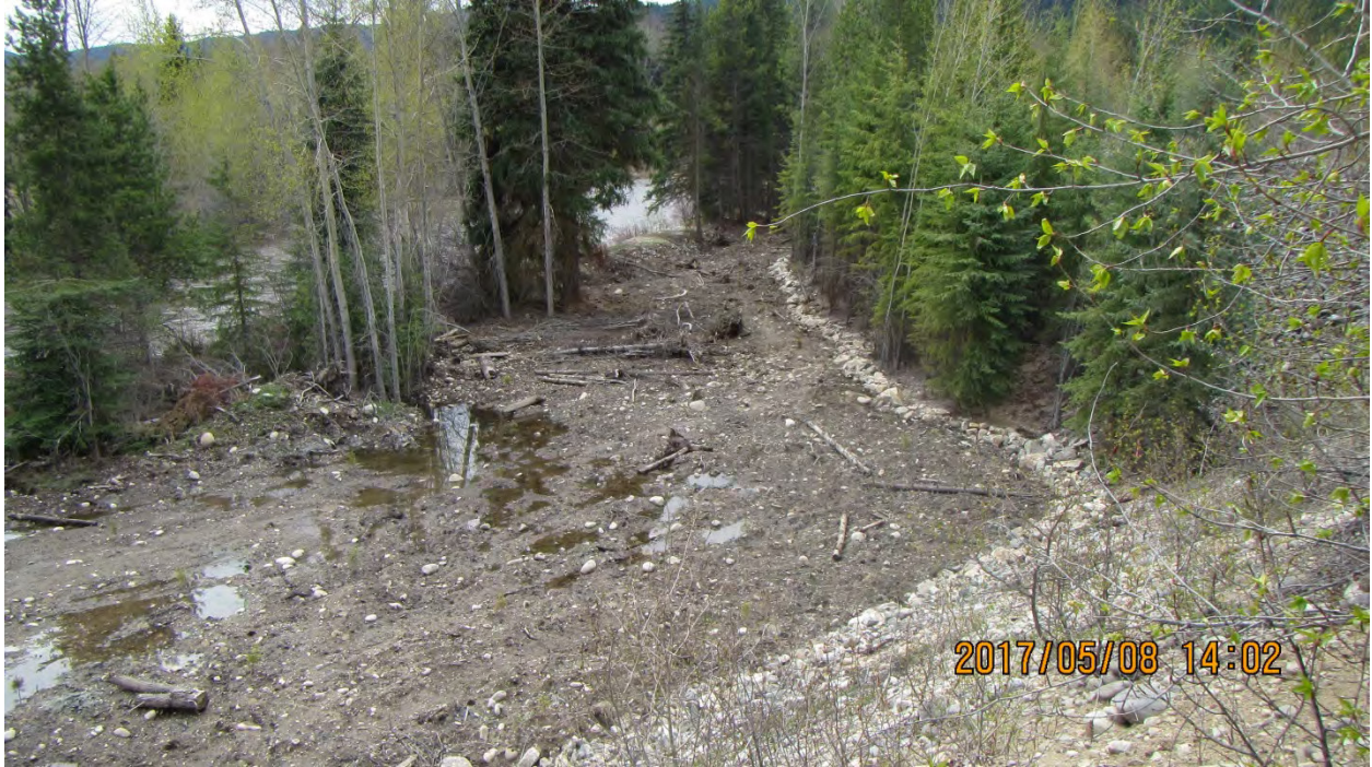
Photo 5 Exposed riprap along cell 5
