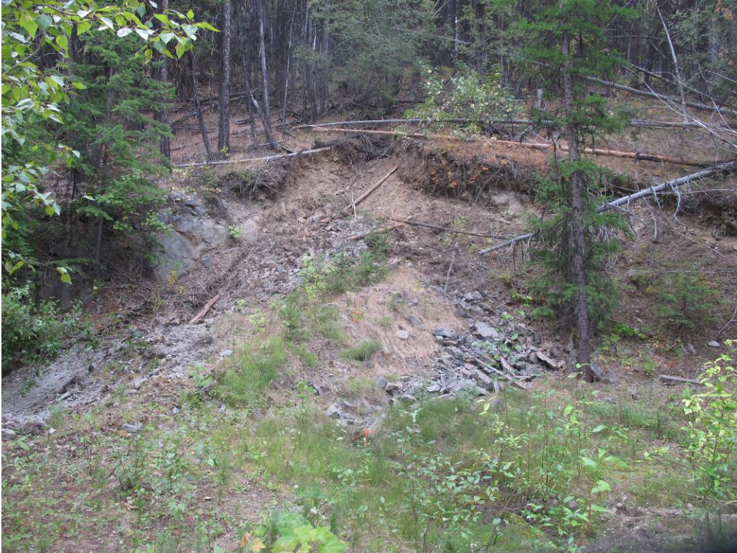
Photo 7: Completed backfill of mine adit
