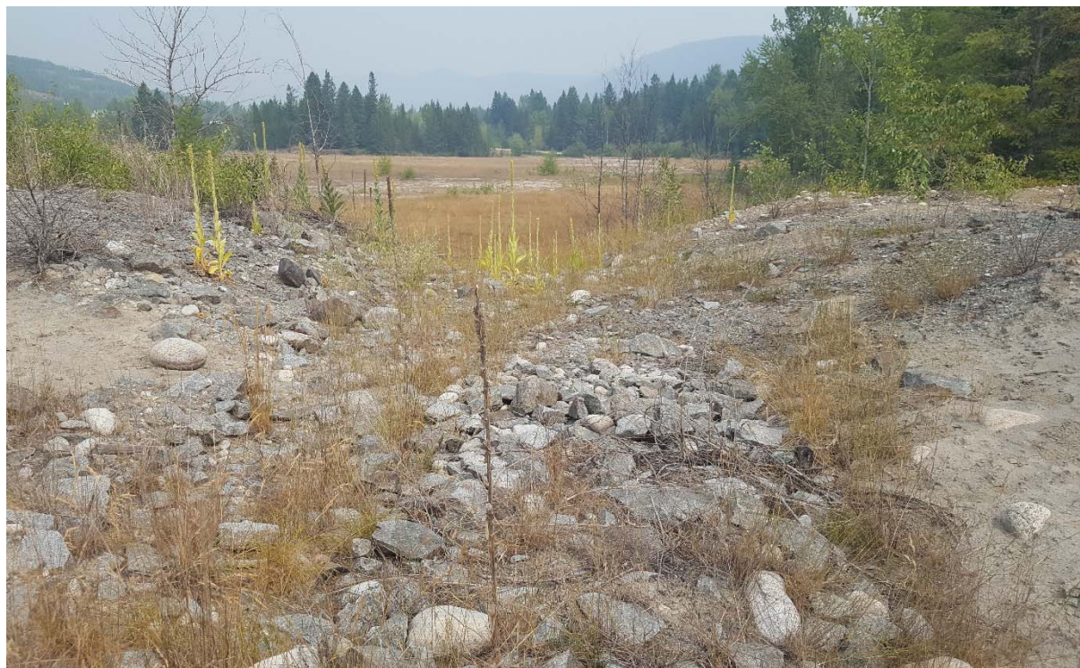
Photograph 22: South TSF, spillway between Cell 4 and Cell 3, looking north. 8 August 2017.
