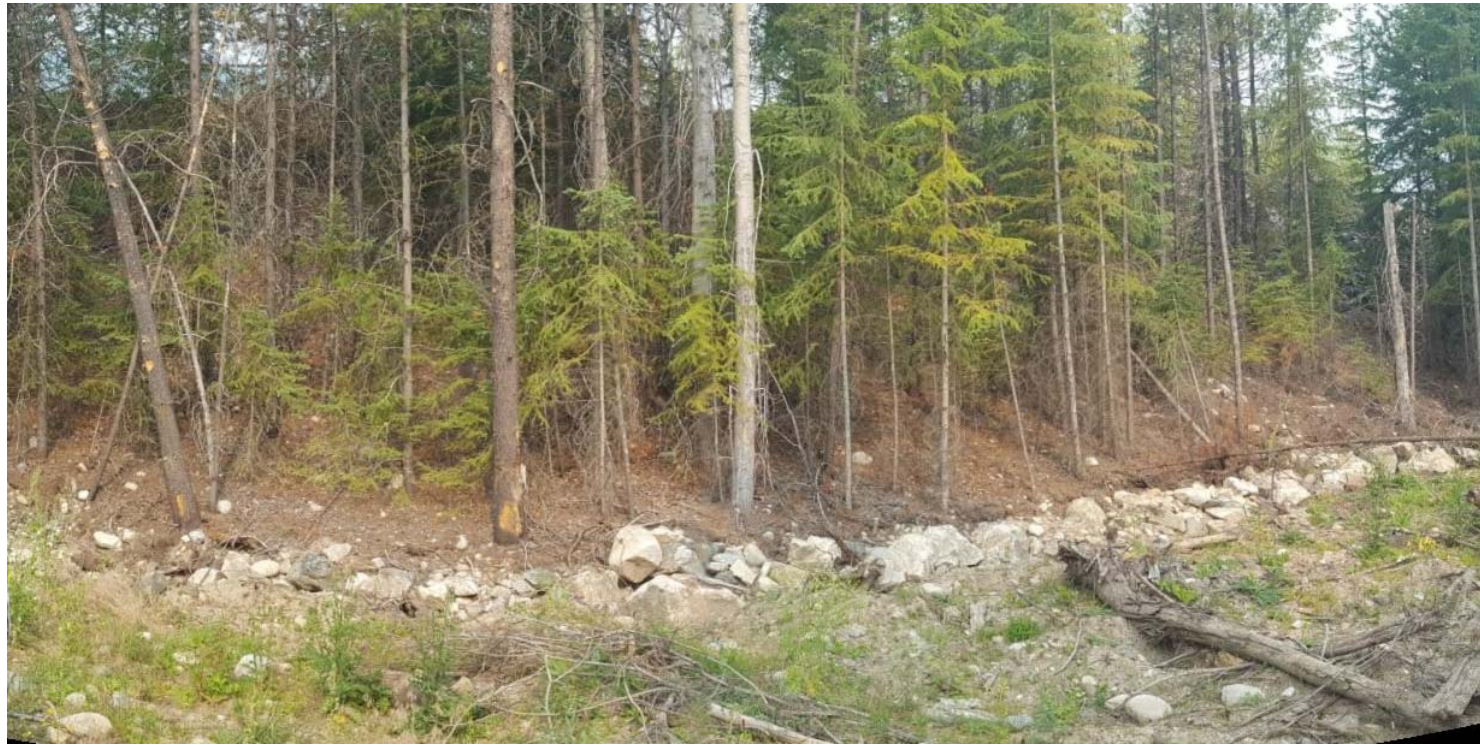
Photograph 12: South TSF, Cell 5, buried riprap at toe of downstream slope, looking northwest. 8 August 2017.
