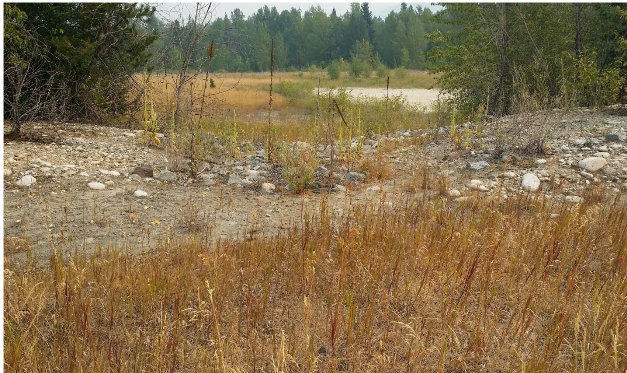
Photograph 16: South TSF, internal spillway between Cell 5 and Cell 4, looking northeast. 8 August 2017.
