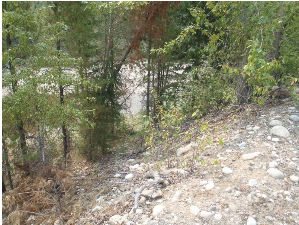
Photograph 9: South TSF, Cell 5, downstream dam slope, looking south. 8 August 2017.
