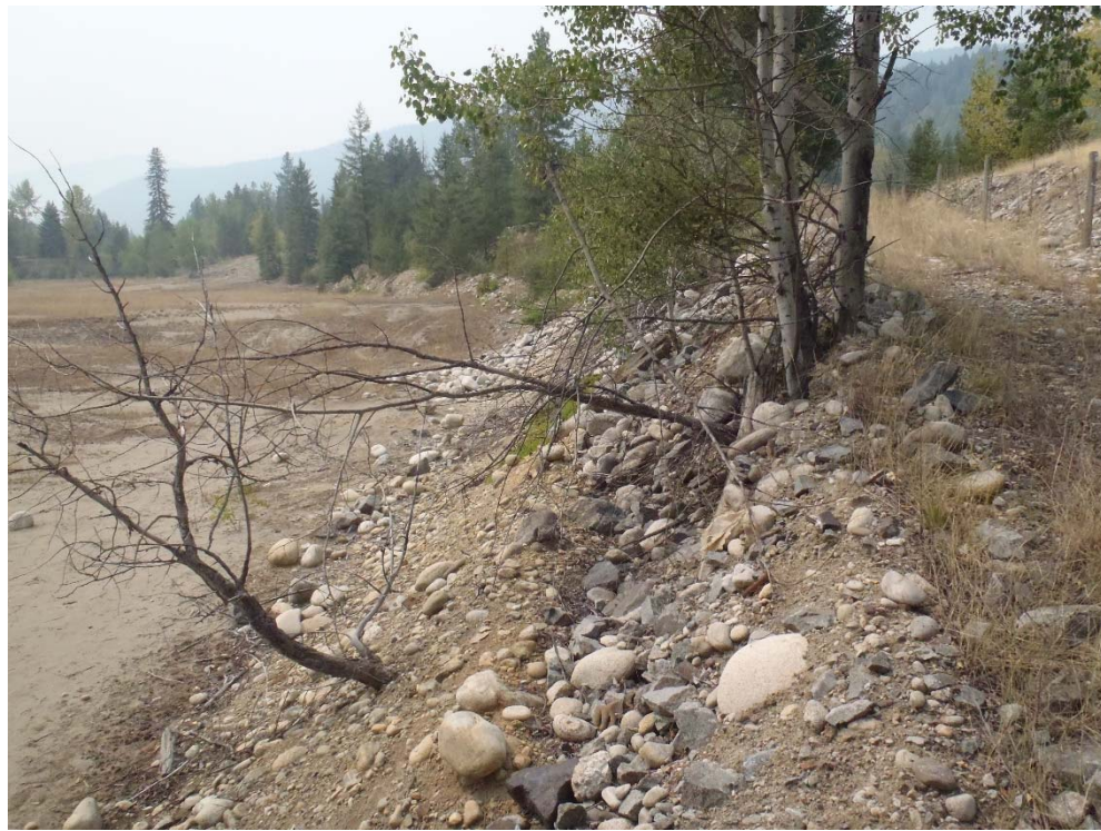
Photograph 31: South TSF, Cell 3, west side of facility upstream slope, looking southwest. 8 August 2017.
