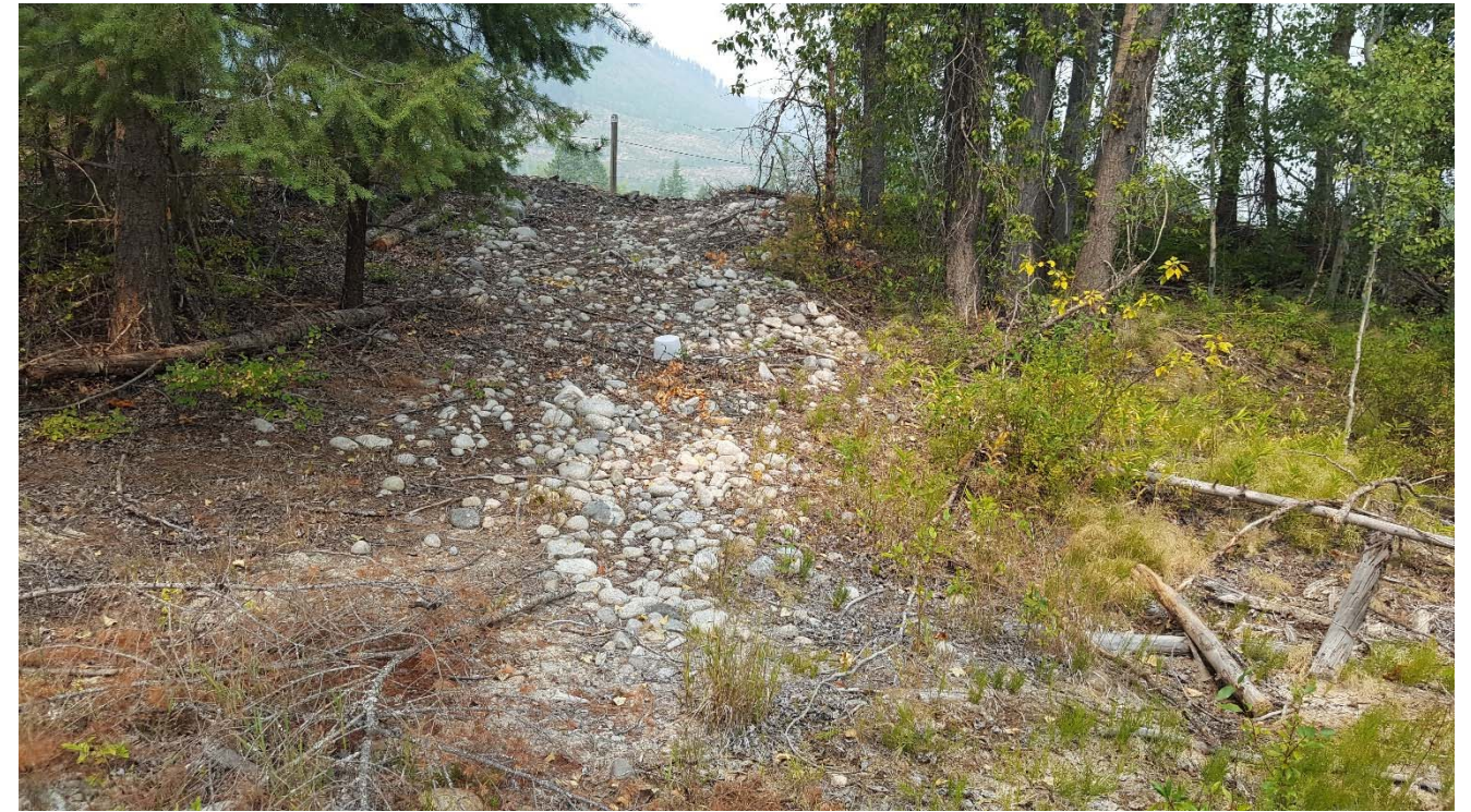
Photograph 28: South TSF, Cell 3, spillway from Cell 3, looking west from downstream toe area. 8 August 2017.
