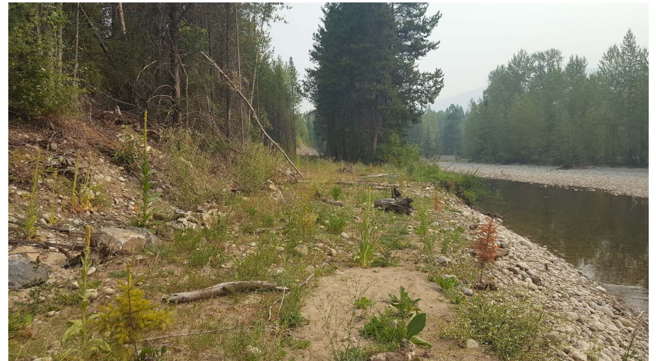
Photograph 14: South TSF, Cell 5, buried riprap at toe of TSF downstream slope, looking northeast. Same location as Photograph 13, low river flow. 8 August 2017.
