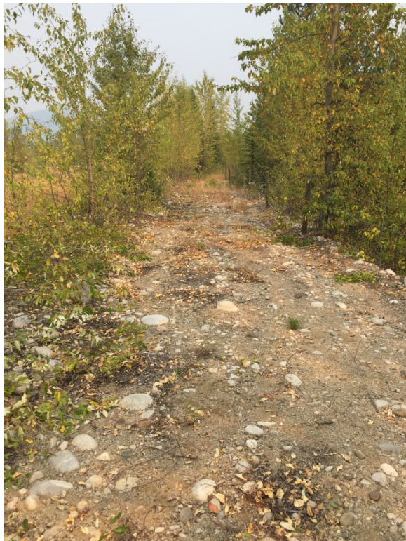
Vegetation on Cell 5 Dike Removed
