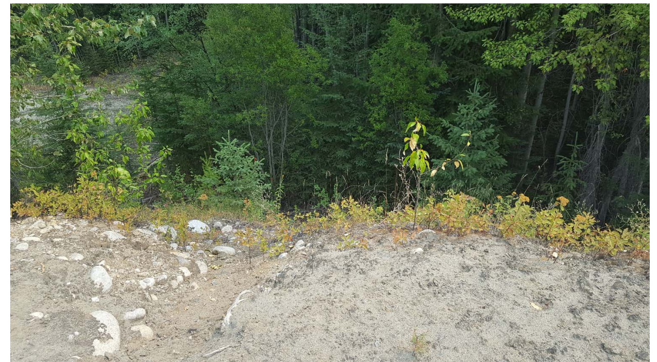
Photograph 20: South TSF, Cell 4, tailings on crest of dam, looking east. 8 August 2017.
