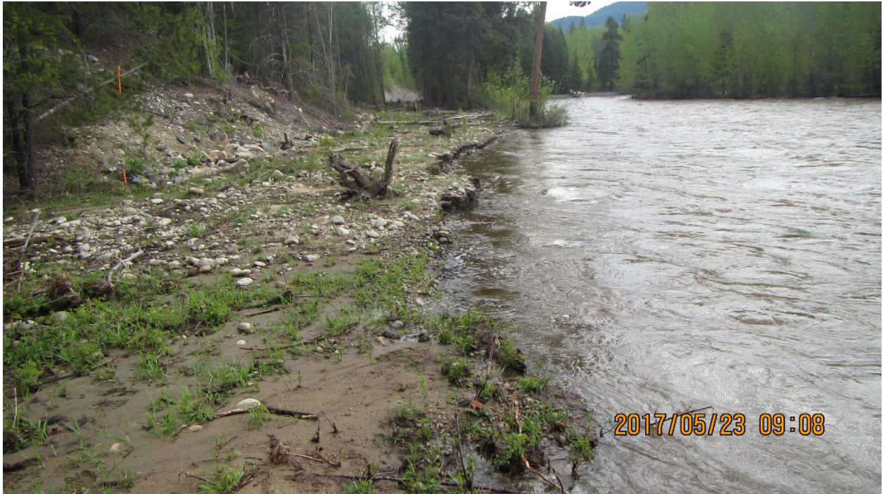
Eroded River bank SE corner of cell 5
