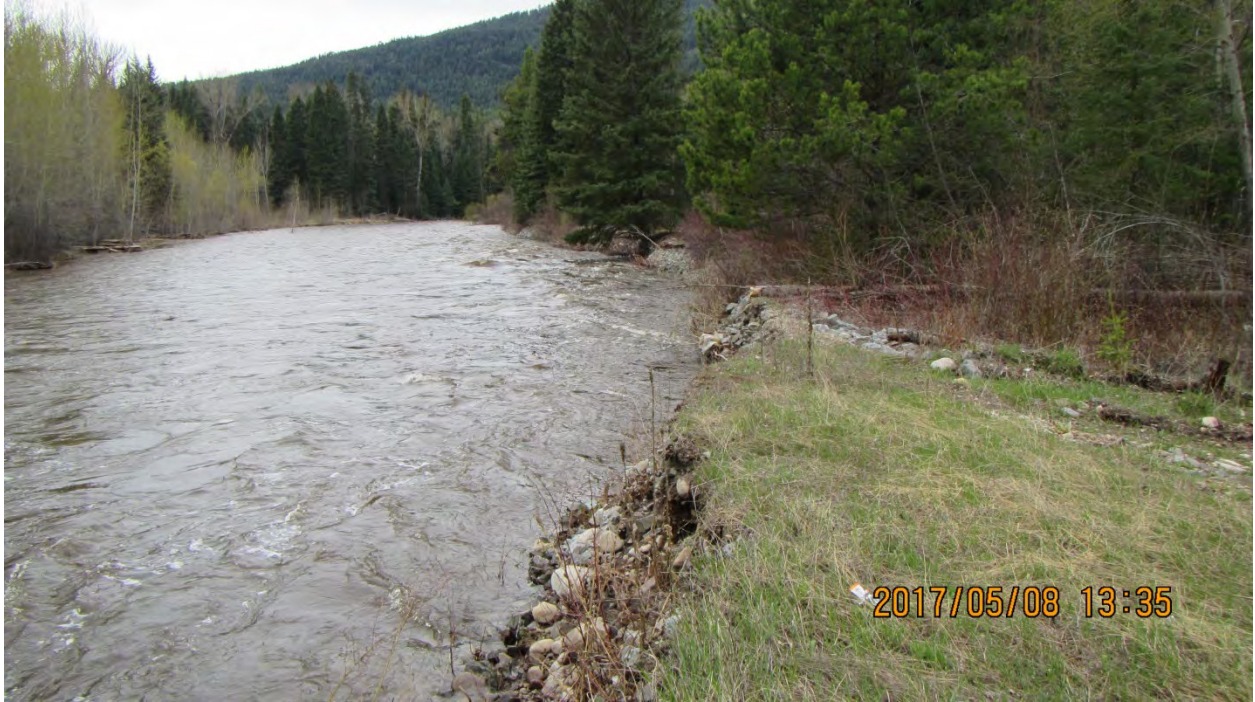
Photo 1 Deterioration in berm between WKR and Cell 4/5
