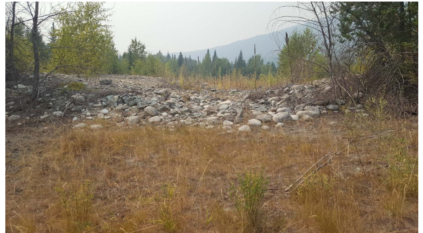
Photograph 17: South TSF, internal spillway between Cell 5 and Cell 4, looking southwest. 8 August 2017.
