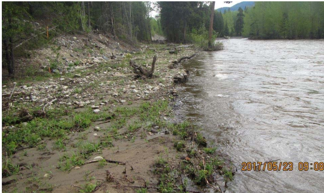
Photograph 13: South TSF, Cell 5, buried riprap at toe of TSF downstream slope during May 2017 high water event, looking northeast. 23 May 2017. Photograph provided by Teck.
