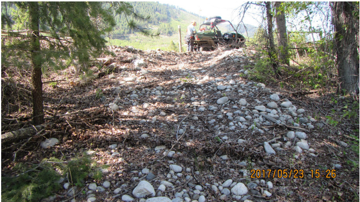
Spillway Debris Removed Cell 3
