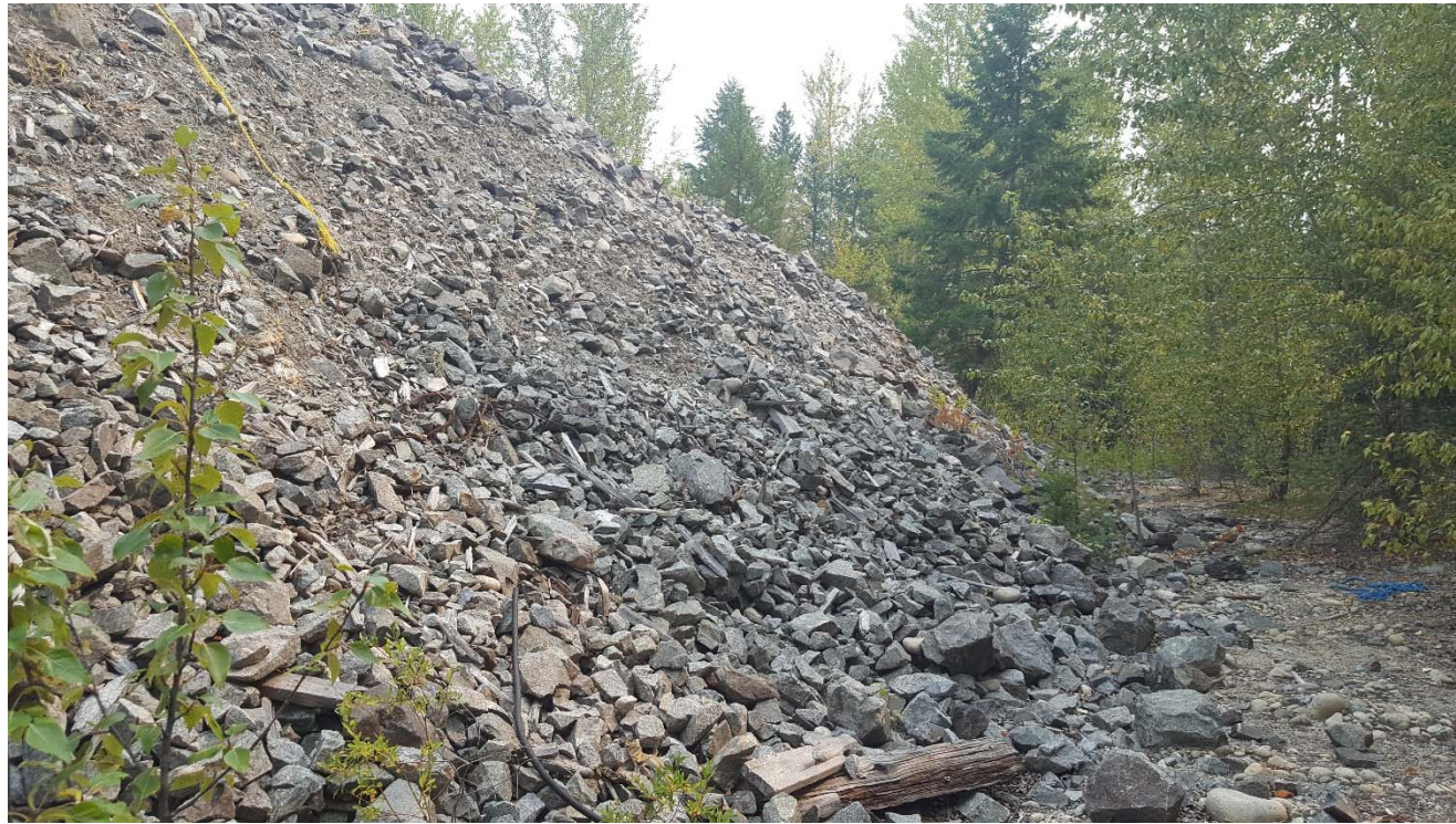
Photograph 15: South TSF, Cell 5, downstream slope consisting of waste rock, looking northeast. 8 August 2017.
