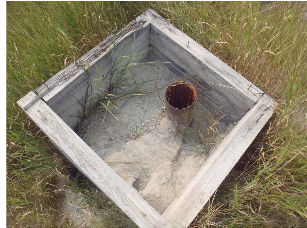
Photograph 10: South TSF, Cell 5, backfilled decant tower, looking east. 8 August 2017.
