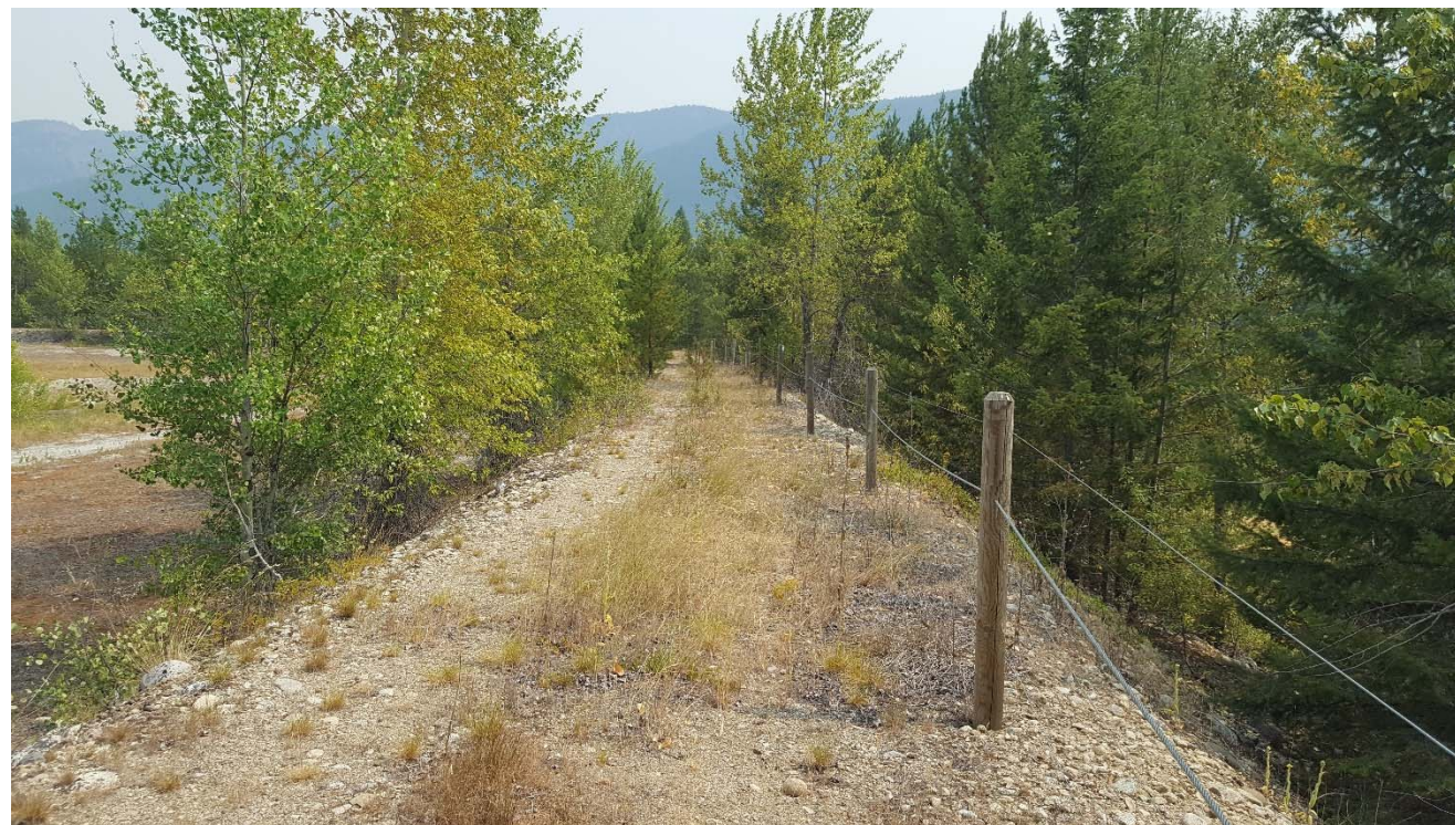
Photograph 43: North TSF, Cell 6, crest of dam on south side of cell, looking east. 8 August 2017.
