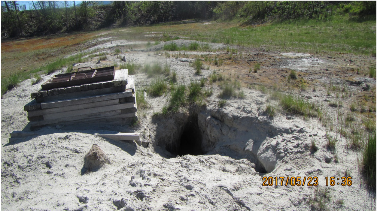
Burrow in Floor of Cell 7
