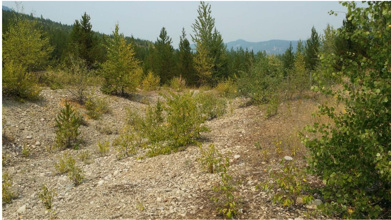
Photograph 47: North TSF, Cell 7, spillway at southwest corner, looking north. 8 August 2017.
