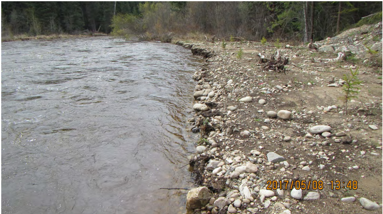
Photo 2 Deterioration in river back, by south corner of Cell 5
