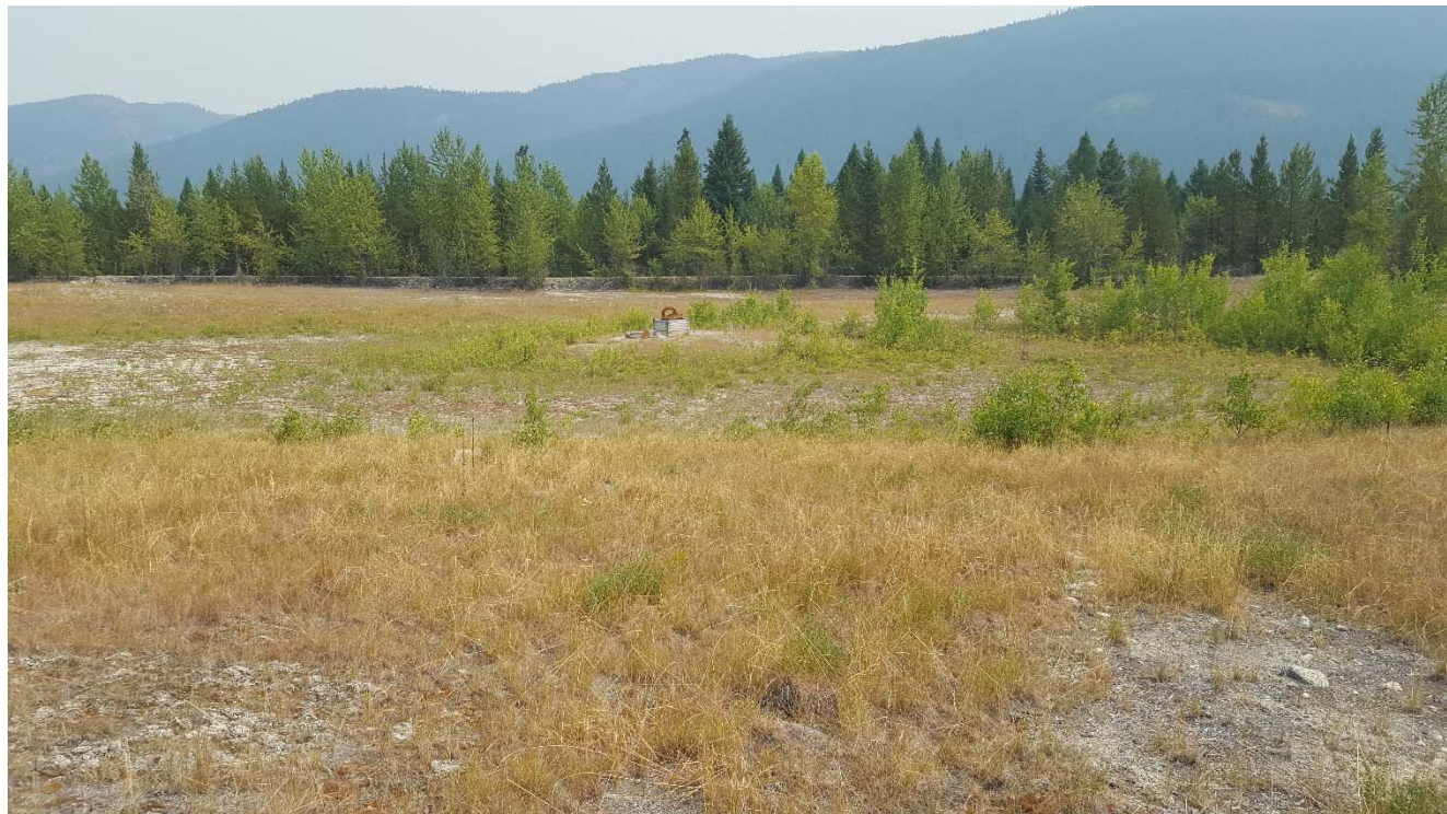
Photograph 39: North TSF, Cell 6, plugged decant tower, looking east. 8 August 2017.
