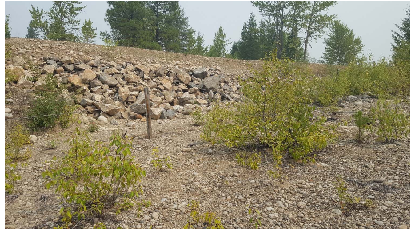
Photograph 6: South TSF, Cell 1, embankment at southeast corner of cell, looking north. 8 August 2017.
