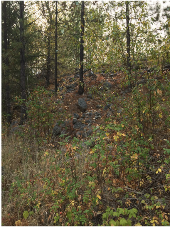
North Downstream Face Cell 7
