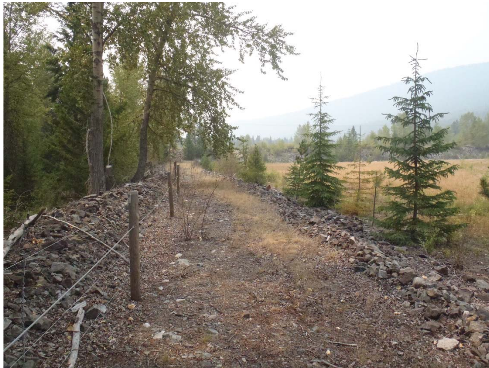
Photograph 29: South TSF, Cell 3, crest of dam on east side of cell, looking south. 8 August 2017.
