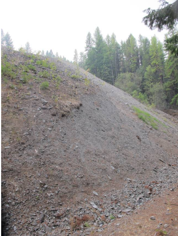
Photo 5: Typical waste rock dump on property
