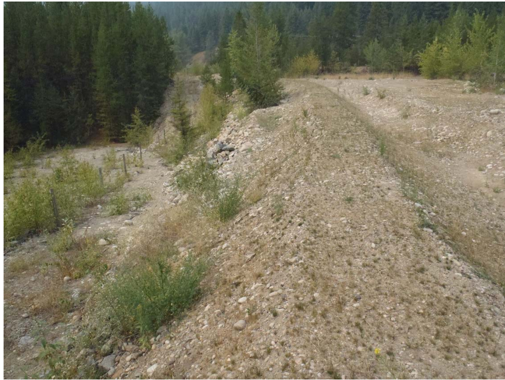
Photograph 5: South TSF, Cell 1, embankment at southeast corner of cell, looking west. 8 August 2017.
