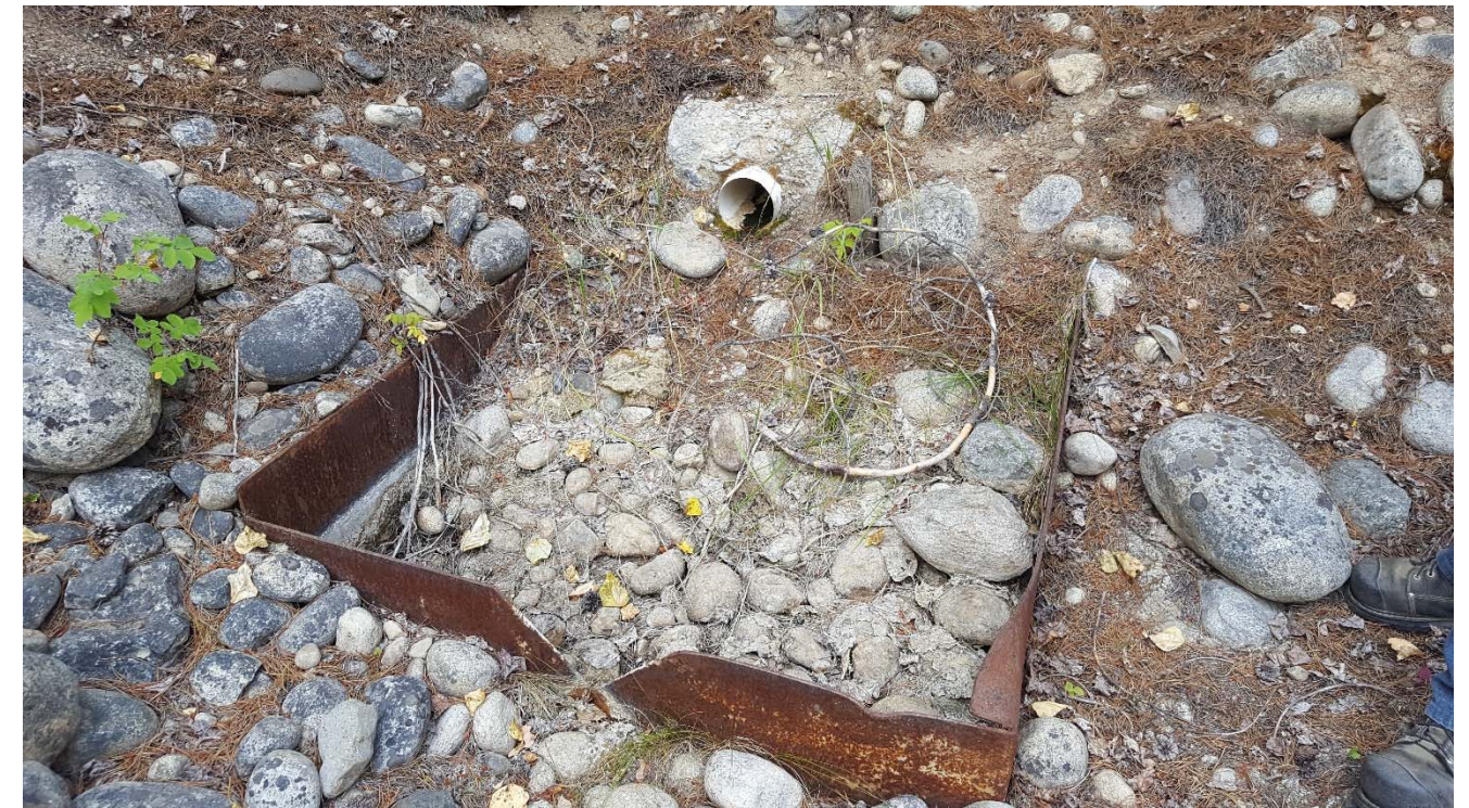
Photograph 42: North TSF, Cell 6, decant outlet at toe of dam, looking northwest. 8 August 2017.
