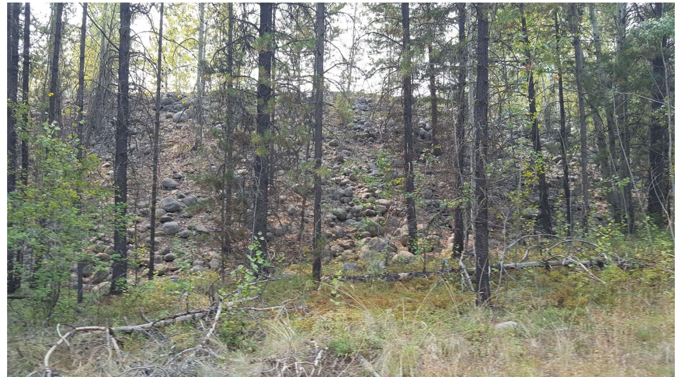
Photograph 40: North TSF, Cell 6, downstream slope and toe, looking south. 8 August 2017.
