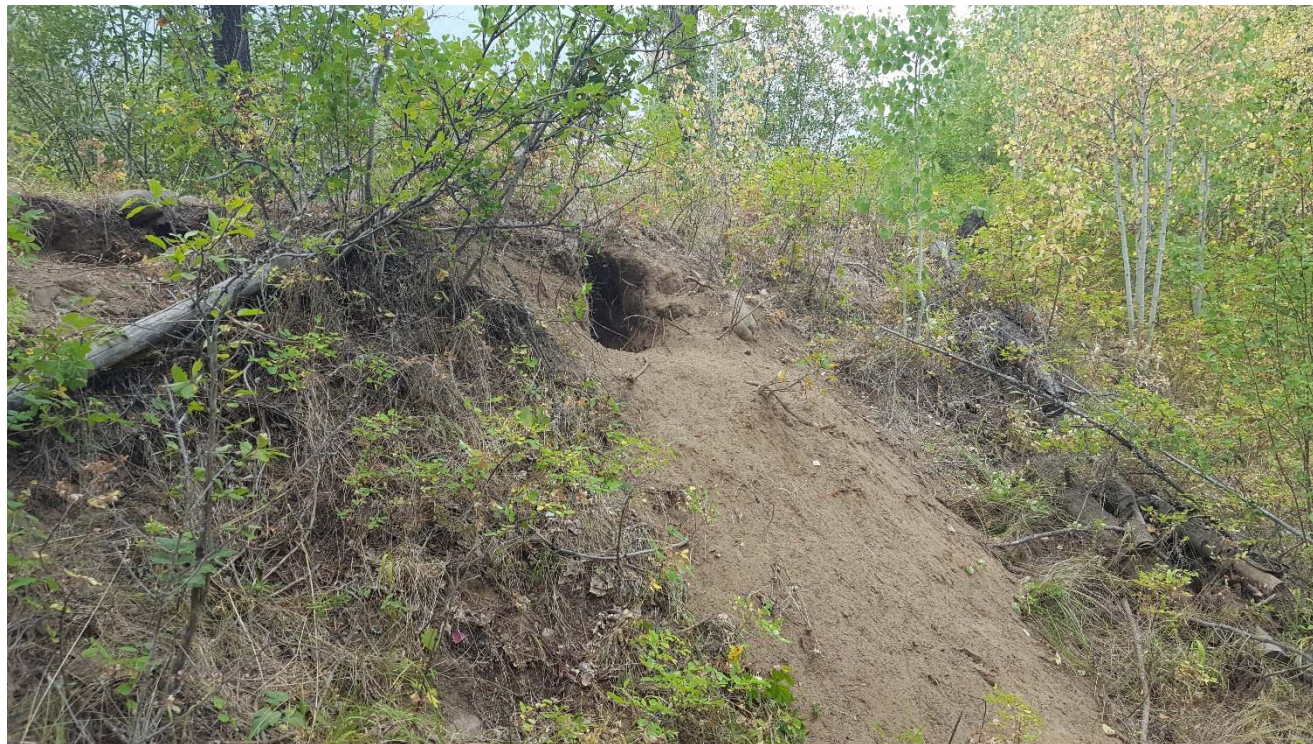
Photograph 33: South TSF, Cell 3, animal burrow in dam on northeast side of cell, looking west. 8 August 2017.
