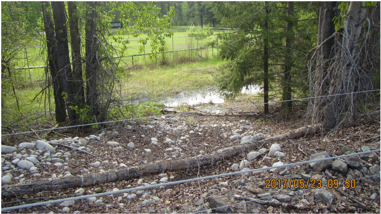
Spillway Debris Cell 3
