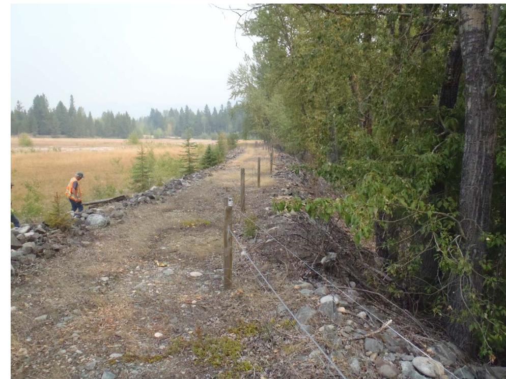
Photograph 26: South TSF, Cell 3, crest of dam on east side of cell, looking northeast. 8 August 2017.
