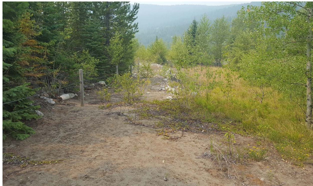
Photograph 19: South TSF, Cell 4, crest of dam, looking south. 8 August 2017.
