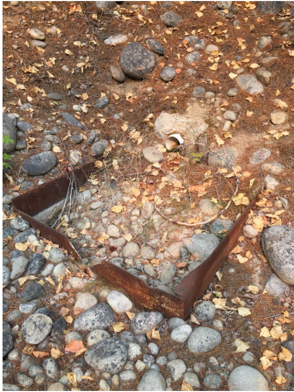
Weir at Decant Outlet Cell 6
