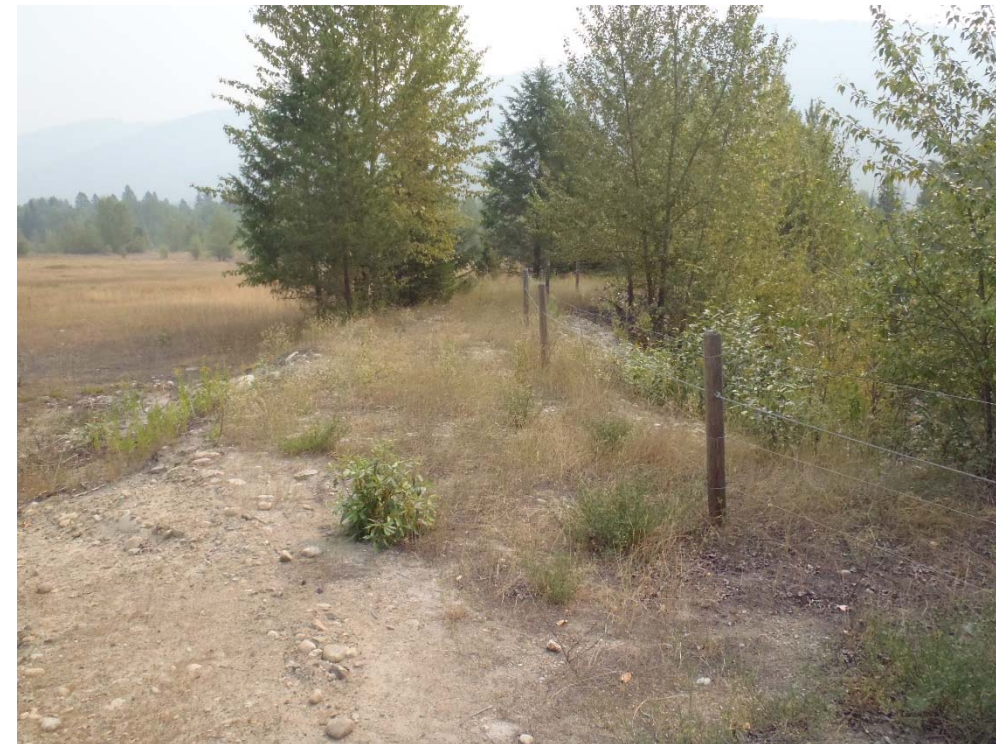
Photograph 8: South TSF, Cell 5, crest on southwest side of dam, looking southeast. 8 August 2017.
