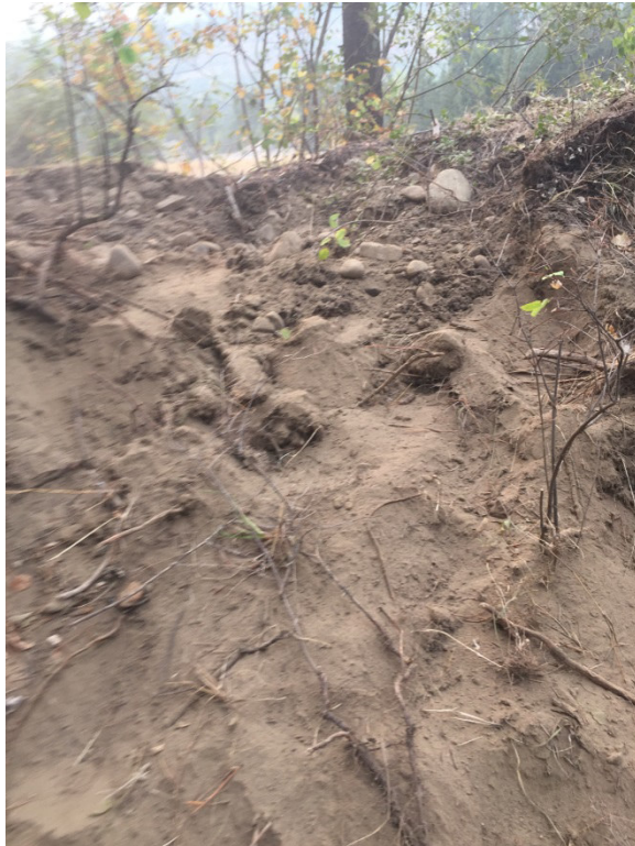
Animal Burrow in Cell 3 Dike Filled In
