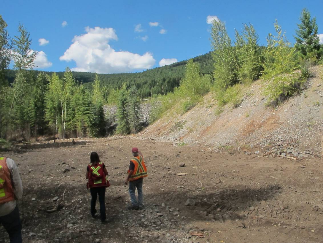
Photo 2: Completion of armoring of toe of Pond 5
