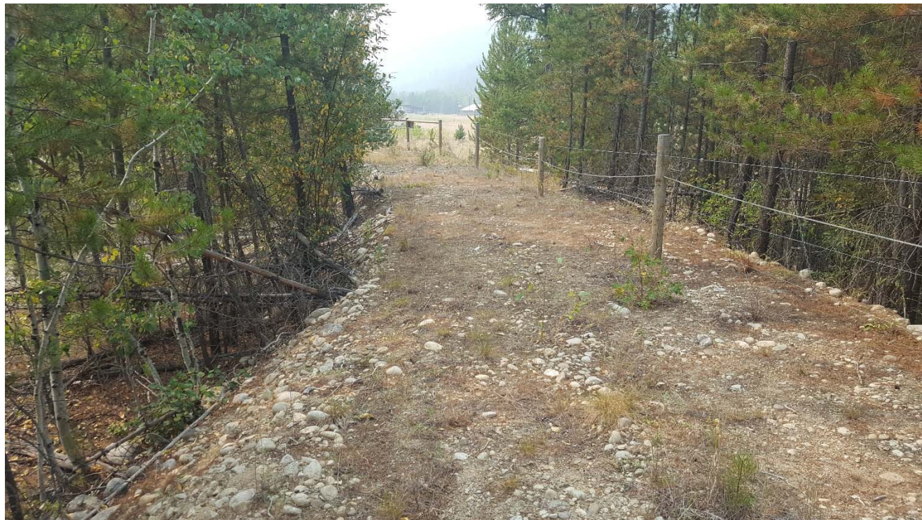
Photograph 3: South TSF, Cell 1, crest of west embankment (access road), looking southwest. 8 August 2017.
