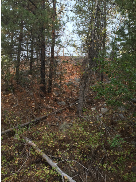
East Downstream Face Cell 6
