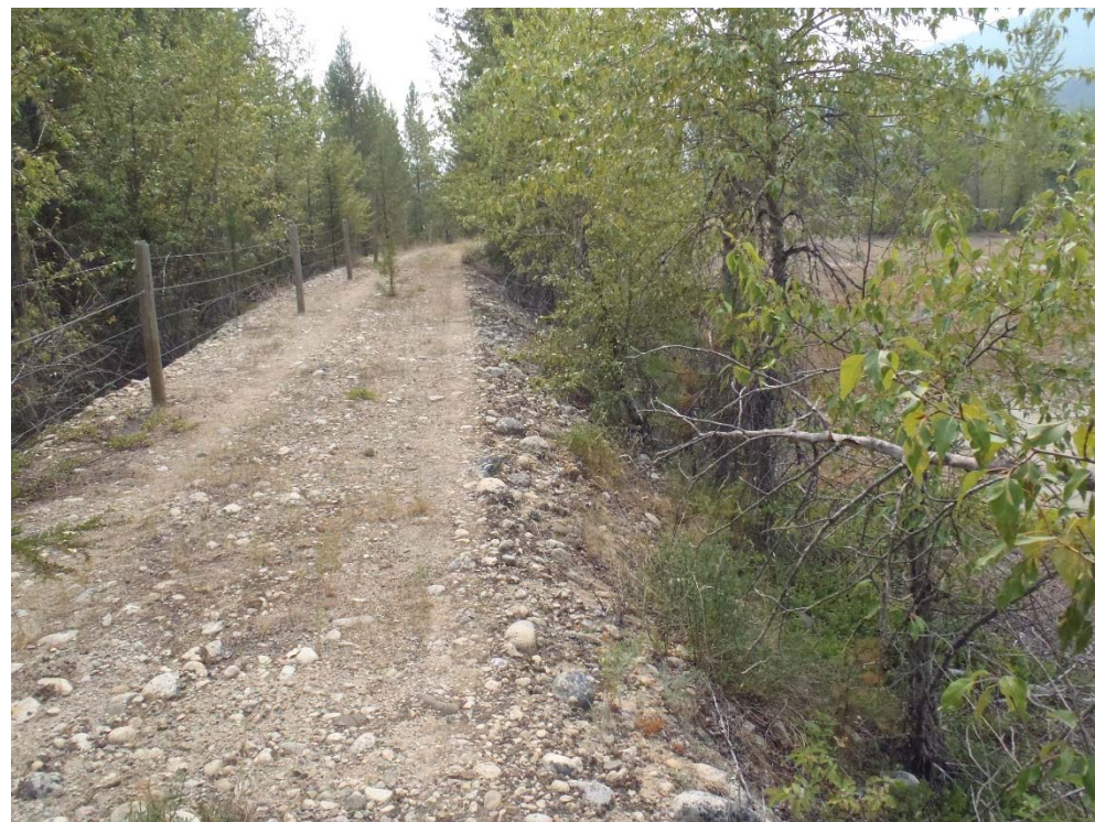
Photograph 35: North TSF, Cell 6, crest and upstream slope of dam, looking south. 8 August 2017.
