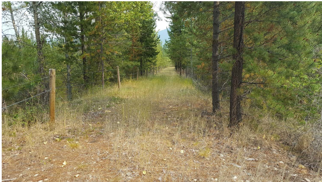
Photograph 45: North TSF, Cell 7, crest of dam on north side of cell, looking east. 8 August 2017.
