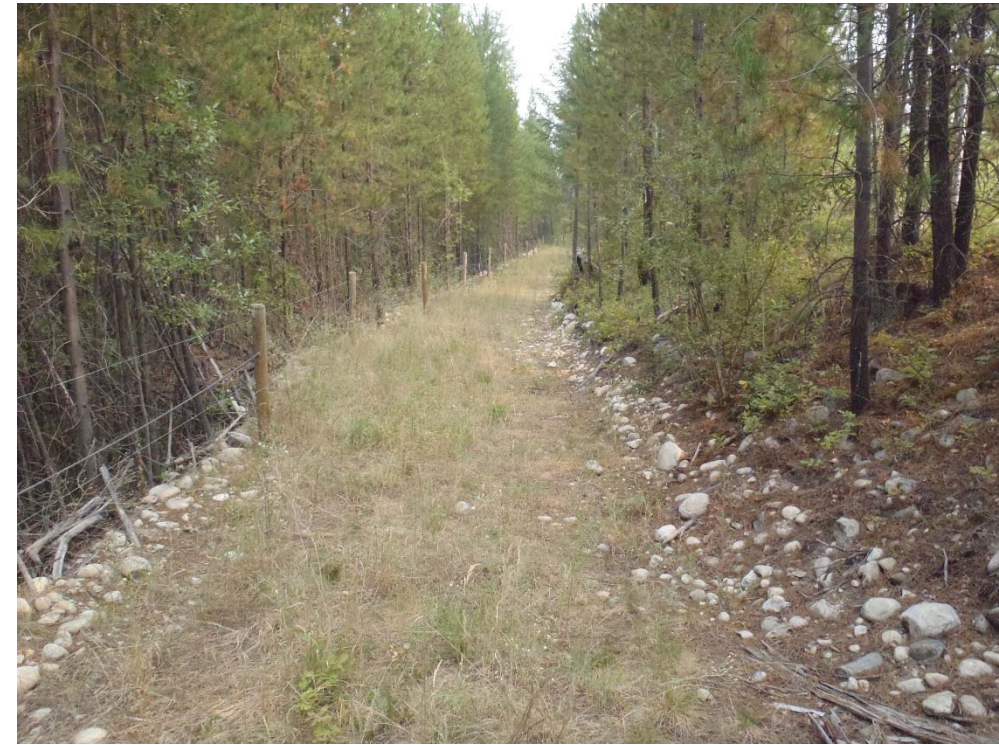
Photograph 2: South TSF, Cell 1, west embankment (access road) with tailings on the right, looking northeast. 8 August 2017.
