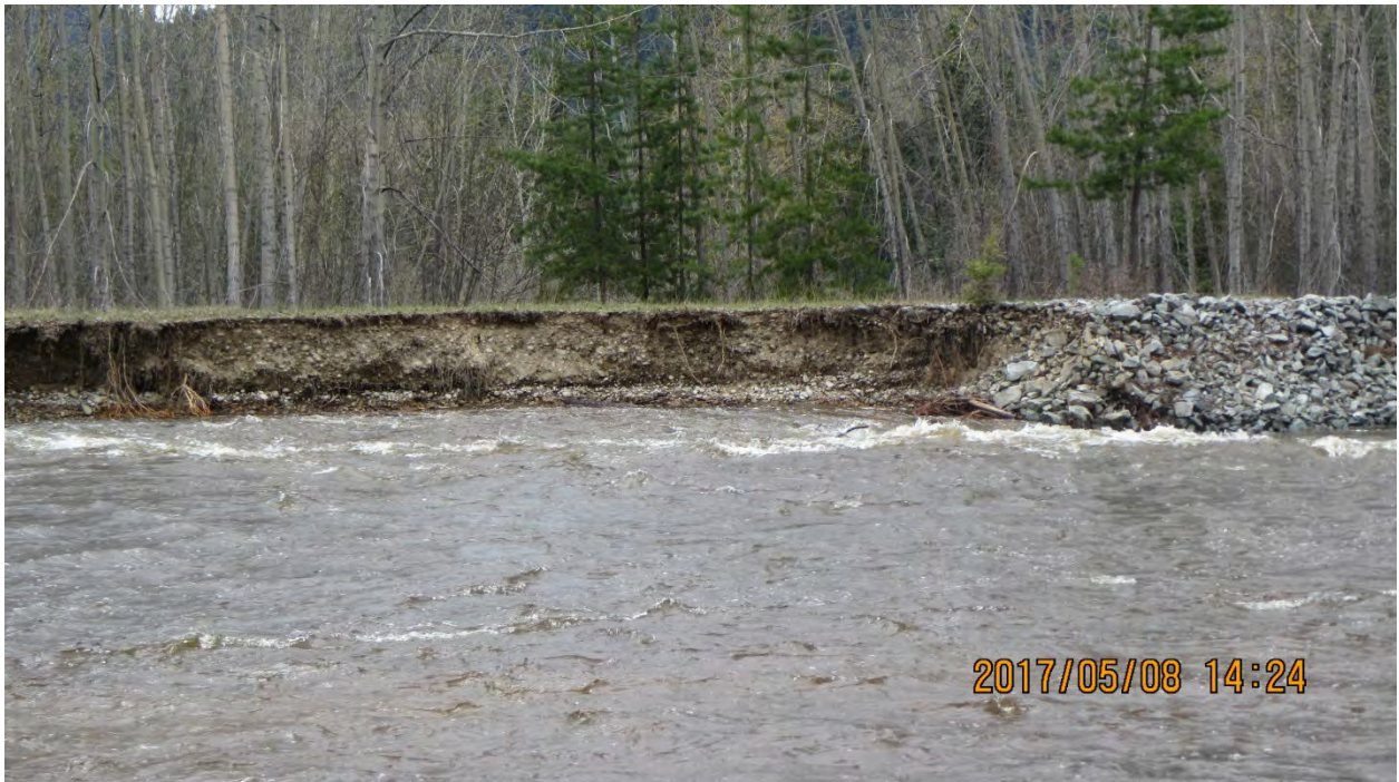
Photo 6 Missing armor and berm section south side of WKR (red hatched section on figure BEA 2017-001)
