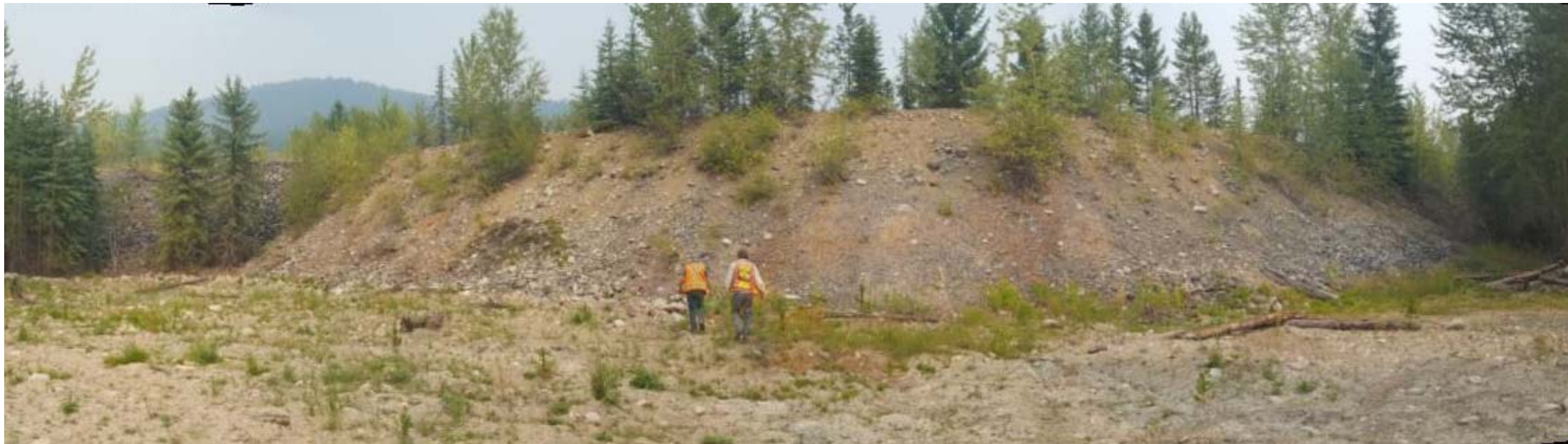
Photograph 21: South TSF, Cell 4, downstream slope and northern extent of buried riprap, looking northwest. 8 August 2017.
