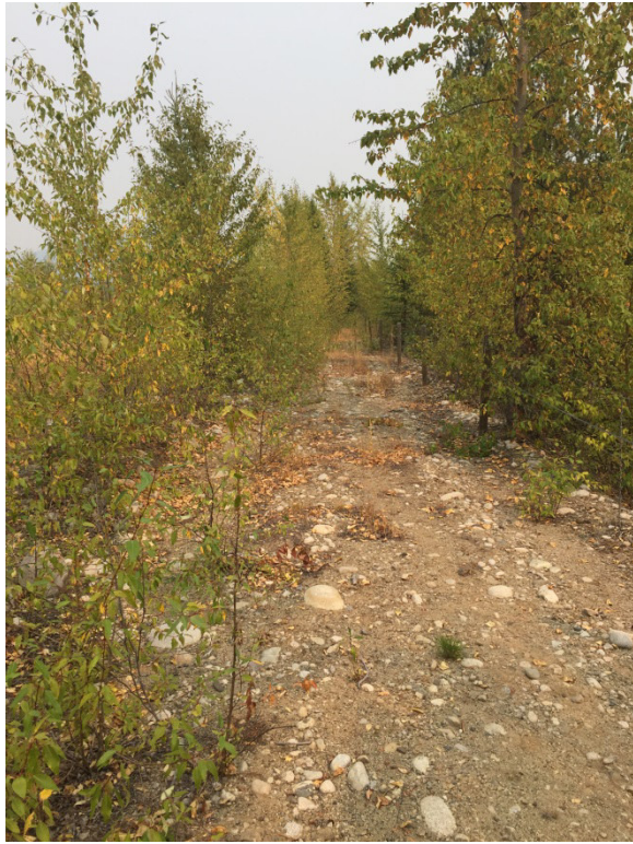
Vegetation on Cell 5 Dike
