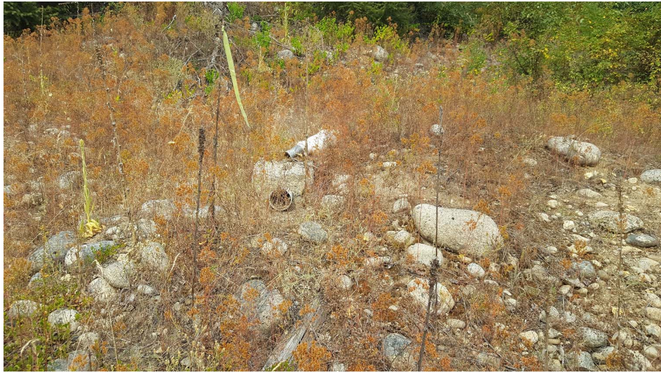
Photograph 51: North TSF, Cell 7, decant outlet at toe of dam, looking north. 8 August 2017.
