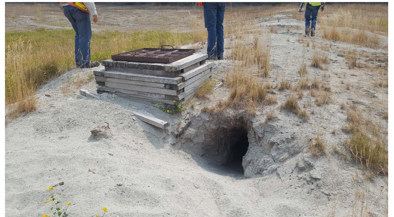
Photograph 50: North TSF, Cell 7, decant tower structure and animal den, looking south. 8 August 2017.
